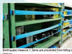
Earthquake measure 1: Items are prevented from falling off shelves.
