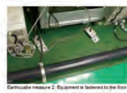
Earthquake measure 2: Equipment is fastened to the floor.
